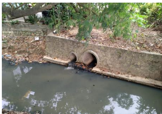
Figure 2. Existing condition of river management in the study area.
