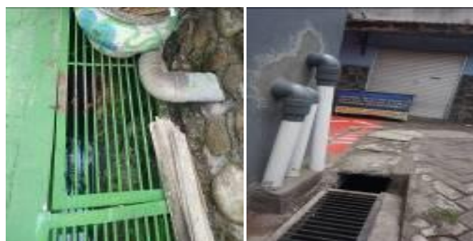
Figure 5. Drainage condition from LED activities.
