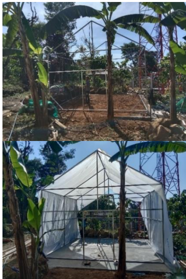
Figure 3. The building process for a coffee drying house
