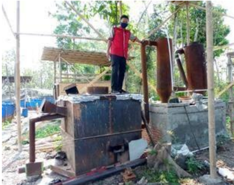
Figure 3. The biomass pellet furnace
