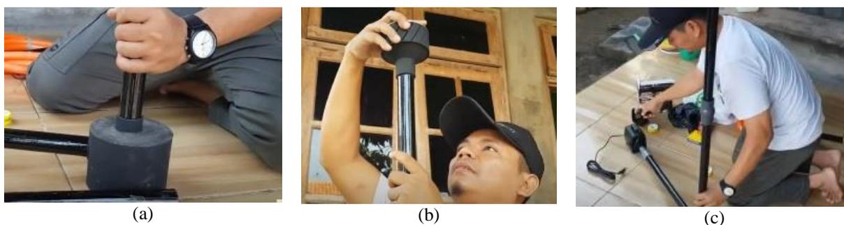
Gambar 9. Pemasangan (a) Vakum draine (b) Skimmer (c) Pompa Air
