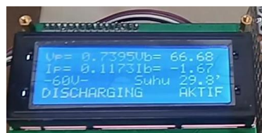
Fig. 20 Discharging Battery Volta 60V
