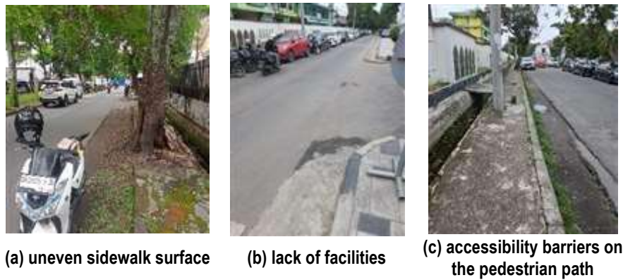
Figure 4. Existing Condition of the Pedestrian Path
