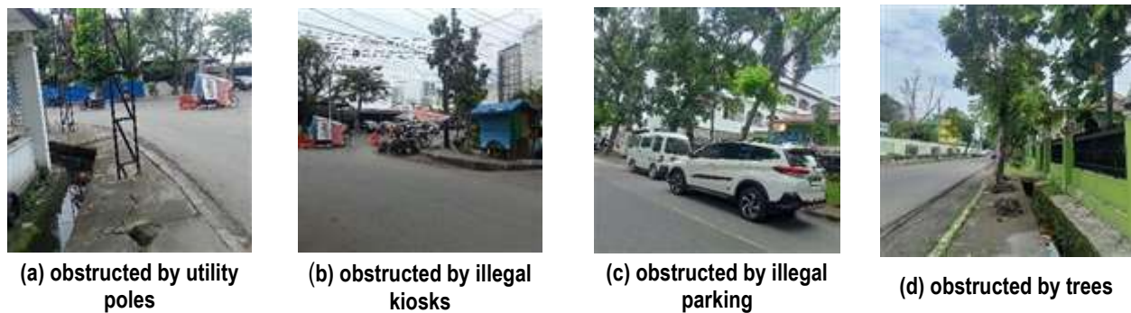
Figure 5. Obstacles on the Pedestrian Path
