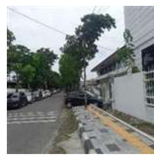
(c) Tactile paving is insufficient
