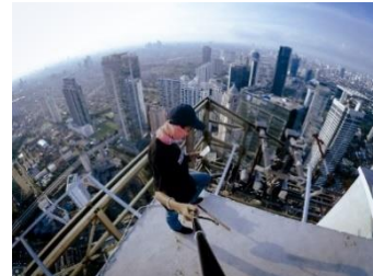
Figure 4. Standing on the edge of a construction site of a skyscraper is one of the most common actions performed by many rooftoppers. Such risky action requires strong nerve since the bottom view is the city scape from hundreds of meters above, which can make many people feel giddy.
