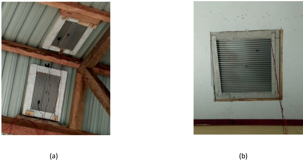
Figure 1. Circuit Placement (a) on Metal Roofing (b) on Ceiling
