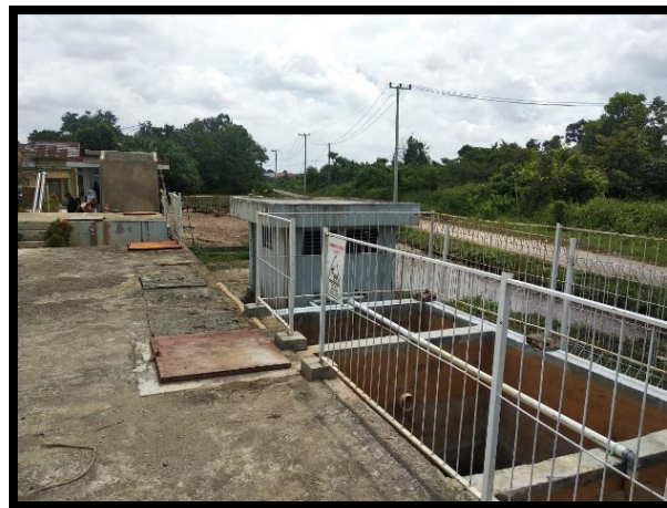
Figure 3. Existing condition of the Cahaya Abadi Housing DWWT
