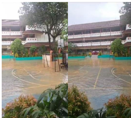
Figure 1. Situation during the flood at the SDN Jatinegara Kaum 03 Jakarta location
