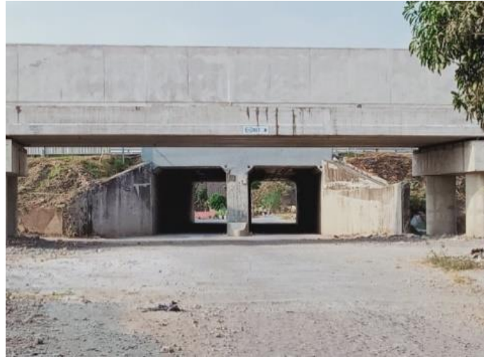
Figure 6. Toll Road Tunnel in Dibal Village
