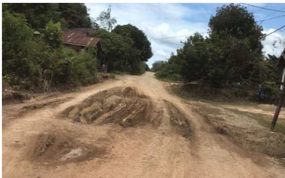
Figure 11. Condition of Road Infrastructure Due to Flood.
