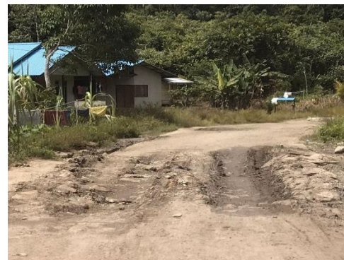
Figure 11. Condition of Road Infrastructure Due to Flood.
