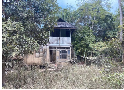
Figure 6. House Affected Flood.
