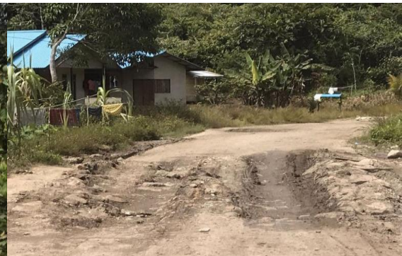
Figure 10. Road infrastructure to the location post-flood research.
