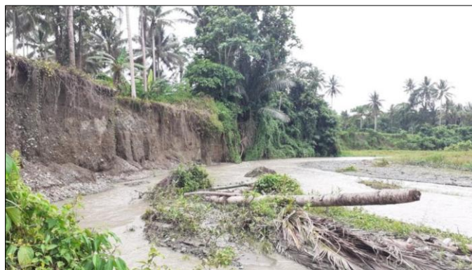
Figure 9. Erosion at The Bend of The River at Tibo Village
