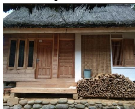
Figure 3. Kampung Naga Traditional House
