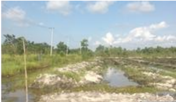
Figure 5. Construction of a Canal in Block 1 of Liang Anggang-KPH Kayu Tangi Source: Field Report, 2021
