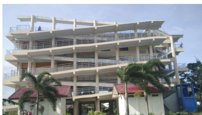
Figure 5. An Escape building at Deah Glumpang Village
