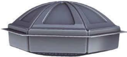
Figure 11. A 1:60 scale replica of the Leipzig wholesale market hall's dome from 1927. (Photograph: 1930 Dischinger)
