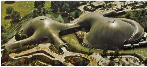
Figure 5: Multihalle at the Bundesgartenschau in Mannheim. Left-hanging chain model (Photo courtesy of Stuttgart's Institute for Lightweight Structures). Correct the completed wooden grid shell. (Photo courtesy of Arup)
