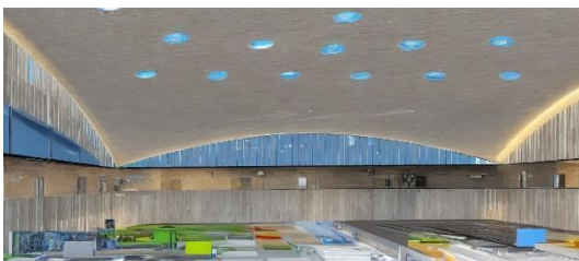
Figure 14. Soho Poultry Marketplace in the British capital, 1963, with a concrete-reinforced shell roof. (Photo by Bill Addis)
