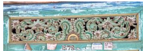
Figure 7. Gebluk Ornaments with Openings for Airflow Entry
