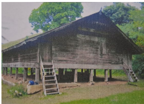
Figure 15. Rear Stair Condition in 2018
