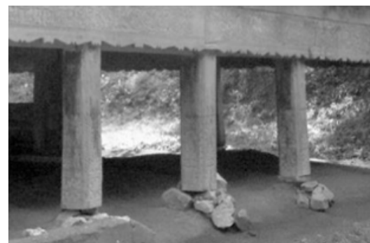
Figure 12. The Foundation of the House in 2015 Source: Ifani, 2015
