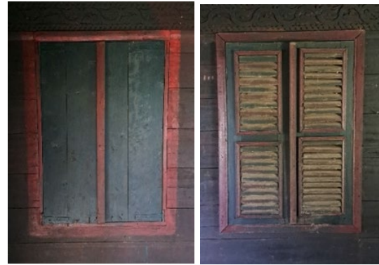
Figure 10. 1st, 2nd, and 4th Room Window (left) 3rd Room Window (right)
