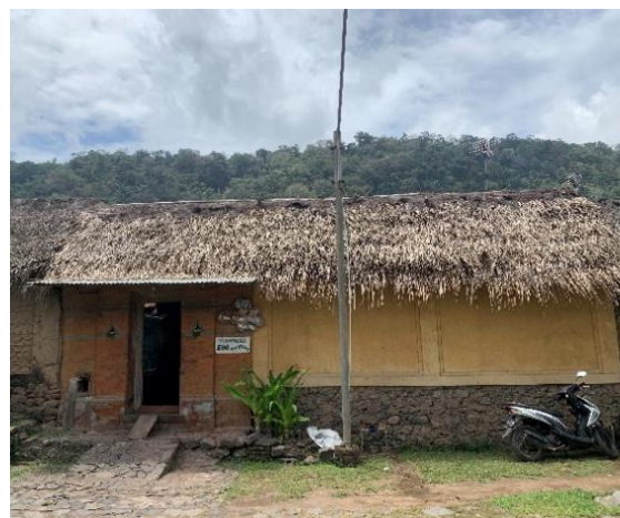
Figure 8. Fasade of the Building at Desa Tenganan, Karangasem (Bali Aga)
