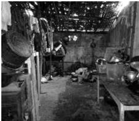
Figure 6. Problematic Air Circulation Condition
