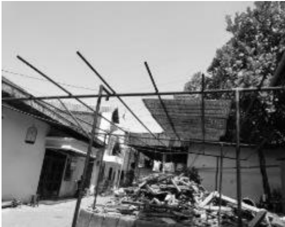
Figure 18. Cracker Drying Place
