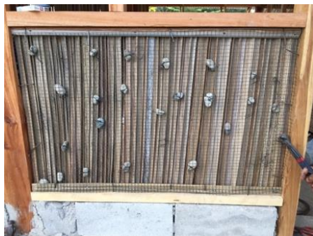
Figure 9. On-site concrete spacer installation on the 2 nd model
