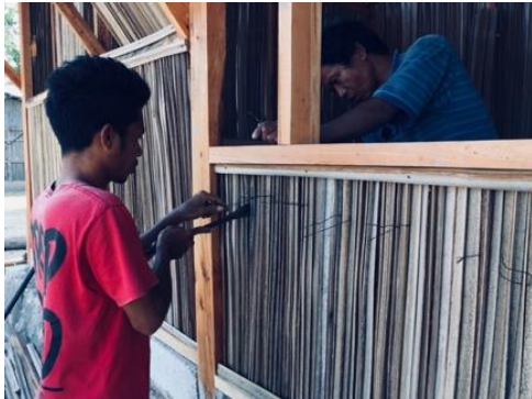
Figure 8. On-site rebar tying wire installation on the 2 nd model
