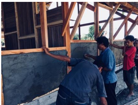
Figure 10. On-site concrete plaster installation of the 2 nd model
