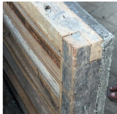
Figure 11. The second model with one-side application of concrete plaster
