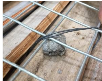
Figure 10. Space between the wire mesh and bebak
