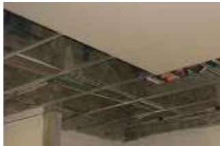
Gambar 5. Plafon Gypsum rangka Hollow Metalfuring (www.google.com)
