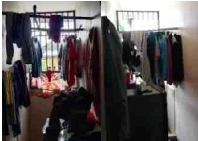
Figure 8. Existing Openings in Residential Unit
