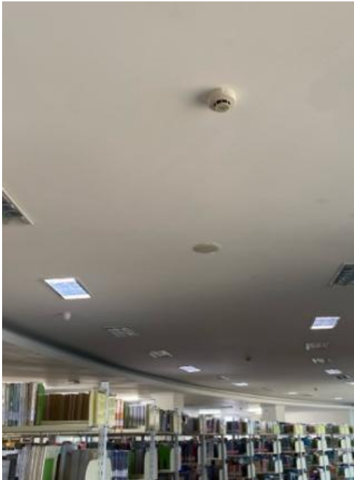
Figure 5. Smoke Detector in Library of UII
