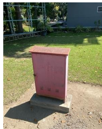
Figure 7. Hydrant in East Library of UII
