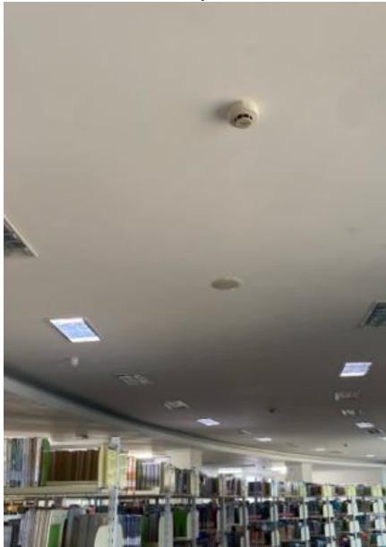
Figure 6. Smoke Detector in Library of UII
