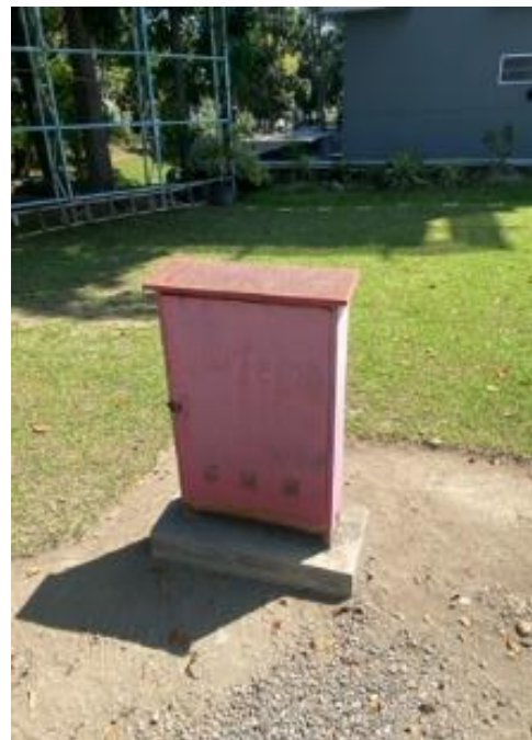
Figure 7. Hydrant in East Library of UII
