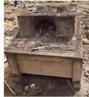
Figure 6. Hawu With Parako Base Part Still Intact During Reconstruction Source: Photograph by Ijad (Local Craftsman/ Palika )
